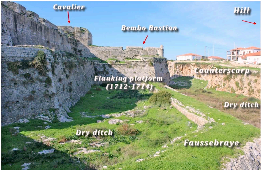
8. Ditch, faussebraye, counterscarp, December 2018.
