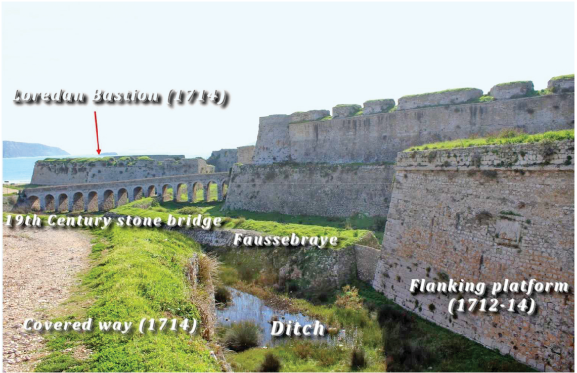
7. Ditch, faussebraye, Loredan Bastion, December 2018.
