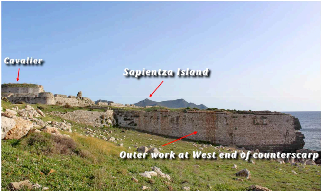
11. Outer work at west end of counterscarp, March 2018.
