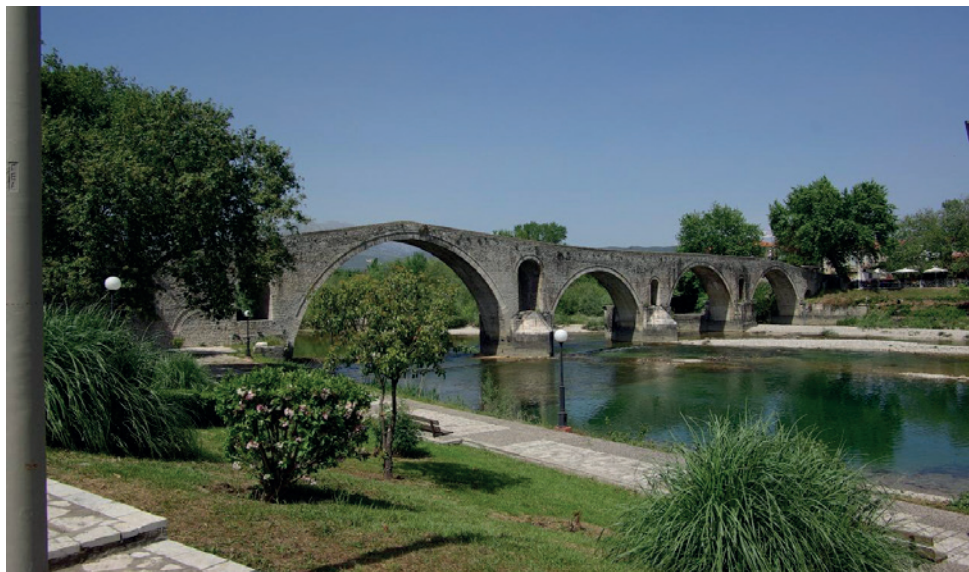
Figure 3. Bridge of Arta.
