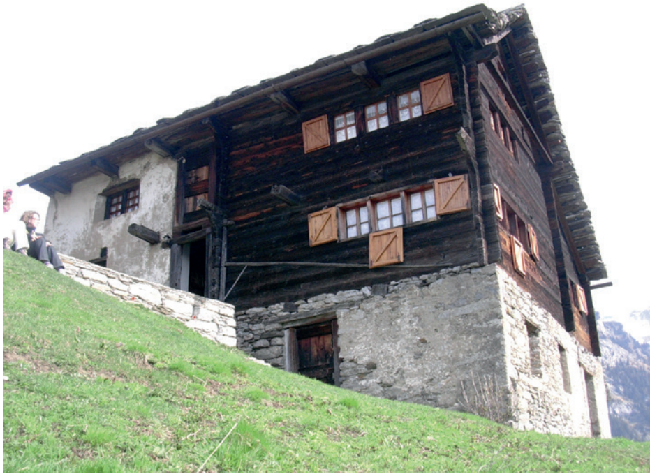
Figure 2. Typical “Blockbau” Walser house (Ossola Valley, 2005).
