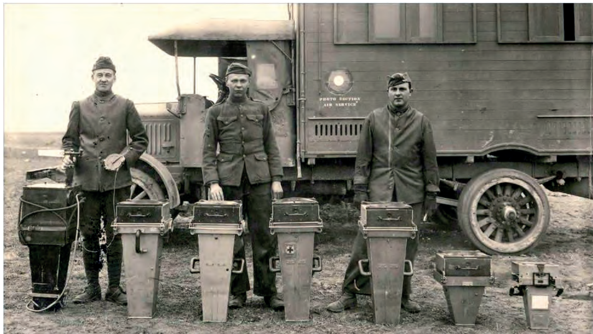
Fig. 5 A British Royal Flying Corps laboratory unit showing all different aero-camera types. (USAFA McDermott Library Special Collections)
